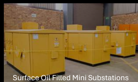
2500kVA Oil Filled Transformer
